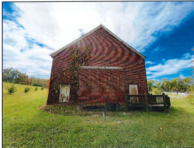
Figure 5: Rear elevation, facing south.
