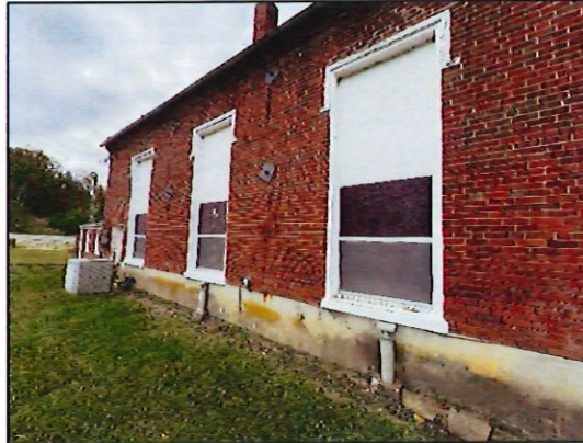
Figure 4: East elevation, facing southwest.
