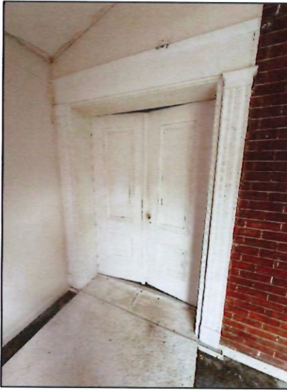
Figure 6: Original double doors at the back of the vestibule, facing north.
