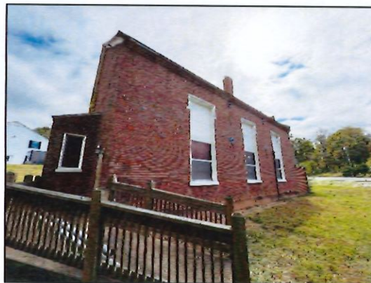
Figure 3: West elevation, facing southeast.
