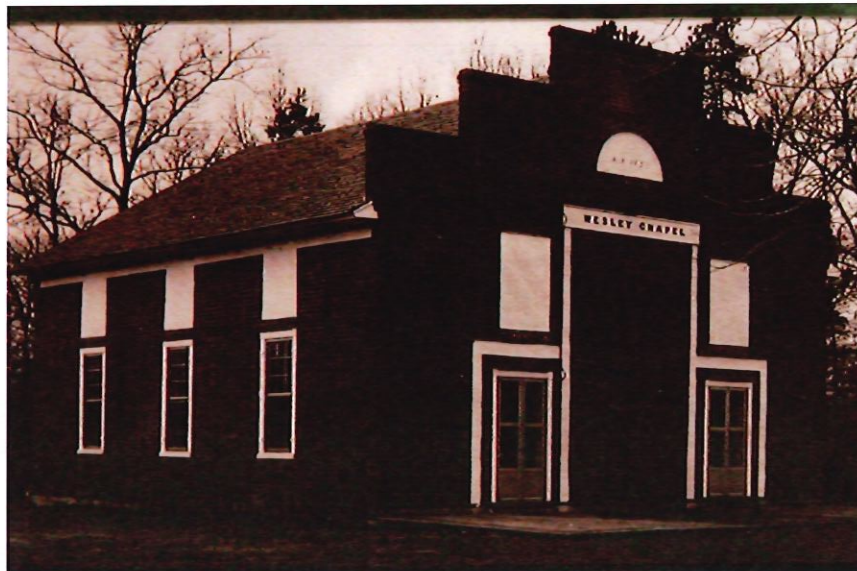
Figure 14. Façade and south elevation of Wesley Chapel, photographer unknown.
